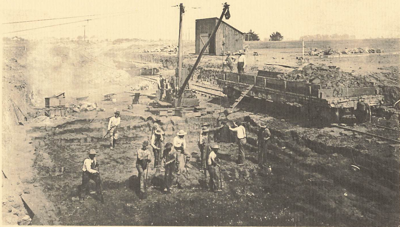
Hot shovel mining operation at the asphalt deposit, 1912. (Photo by George G. McLean).
